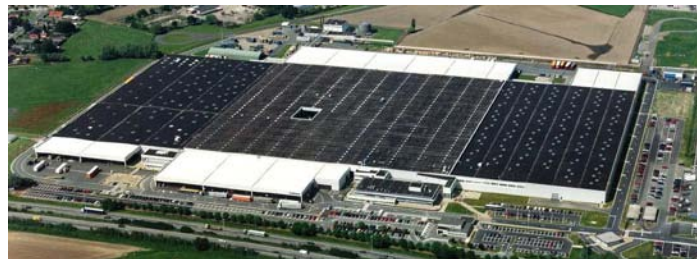
Figure 4.3 Overview of the central warehouse in Ghent, Belgium
