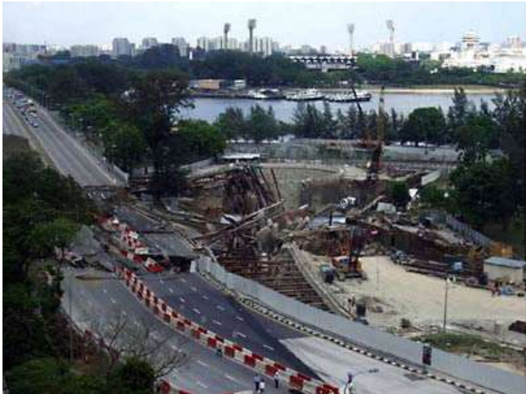
Figure 4 Excavation failure at Nicoll Highway, Singapore, in 2004. This shows the collapse of a retaining wall during the construction of the Singapore MRT. The investigations suggested that the most likely cause of the collapse lay in the design of the retaining wall which proved insufficient to support the earth pressures. This was attributed to the use of an inappropriate soil model which overestimated the soil strength at the site and underestimated the forces on the retaining walls in the excavation.
