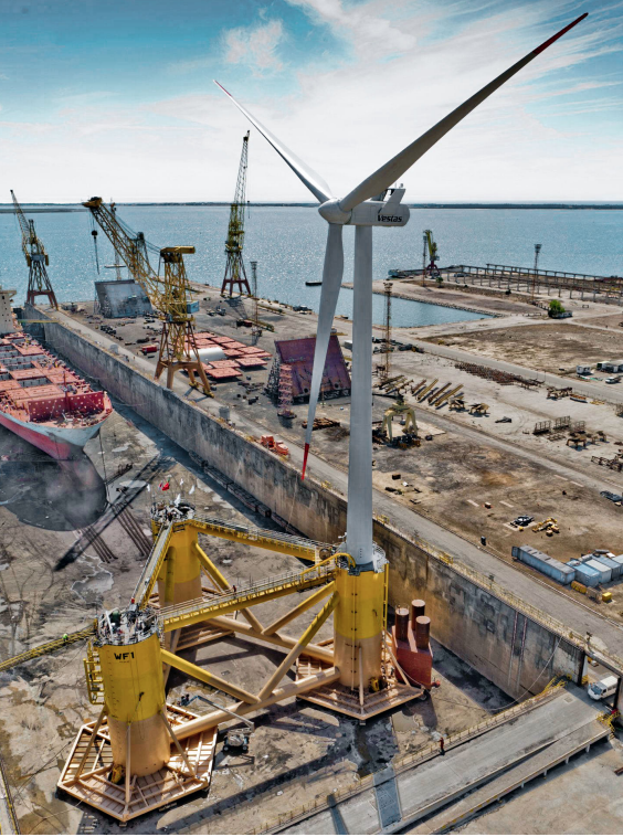
Figure 1: WindFloat assembly in the Mitrena Shipyard near Lisbon. Water entrapment plates are visible at the bottom of the semi-submersible platform's columns. Source: Cermelli (2014), photo courtesy of Principle Power Inc.
