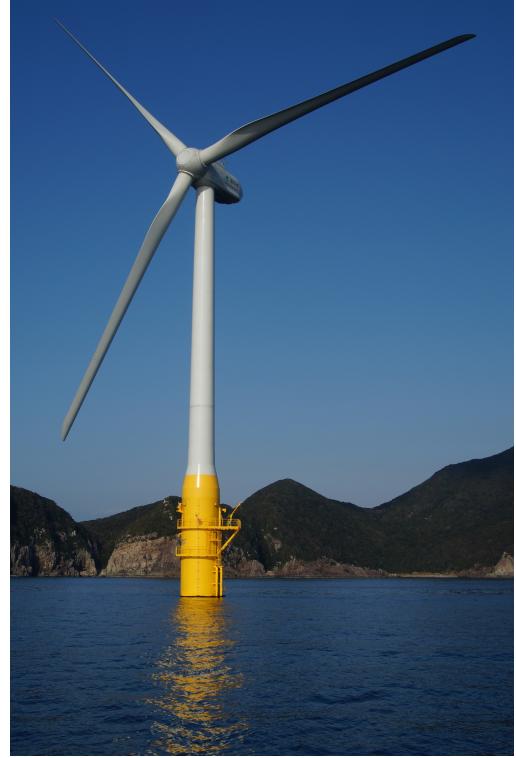
Figure 2: Haen-kaze, the 2 MW floating wind turbine demonstrator sited off Goto in Japan. Photo courtesy of David Ingram.
