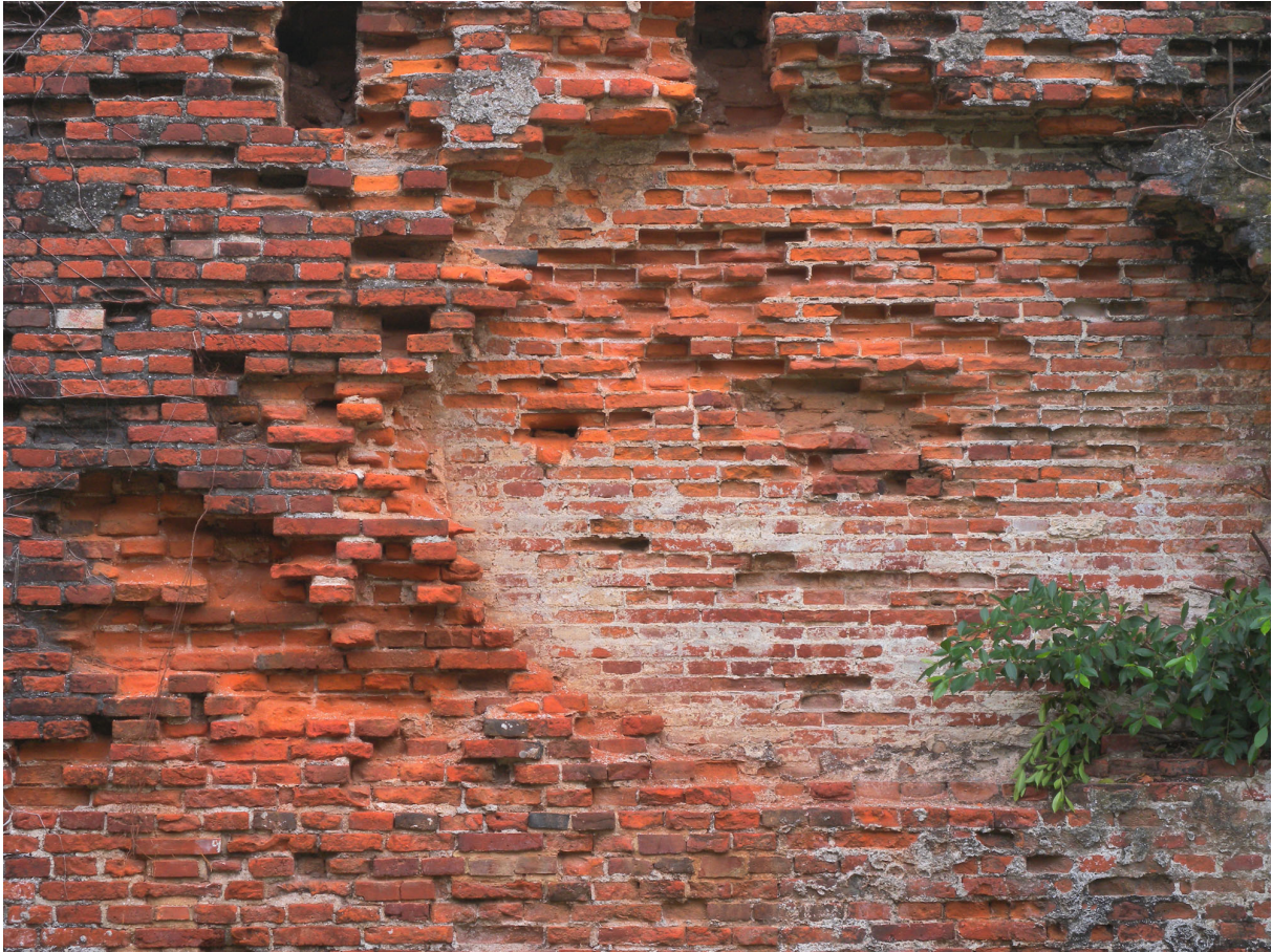
Figure 7. Mixed sizes of bricks, north (inner) elevation, southern remains of outer fort. (Part B in Fig. 3): thicker types facing a thinner-type inner core (author's photo, 2011)
