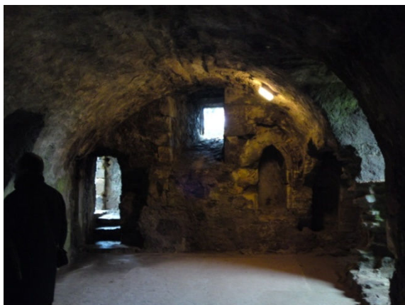
Figure 1. Vaults in Dirleton Castle
