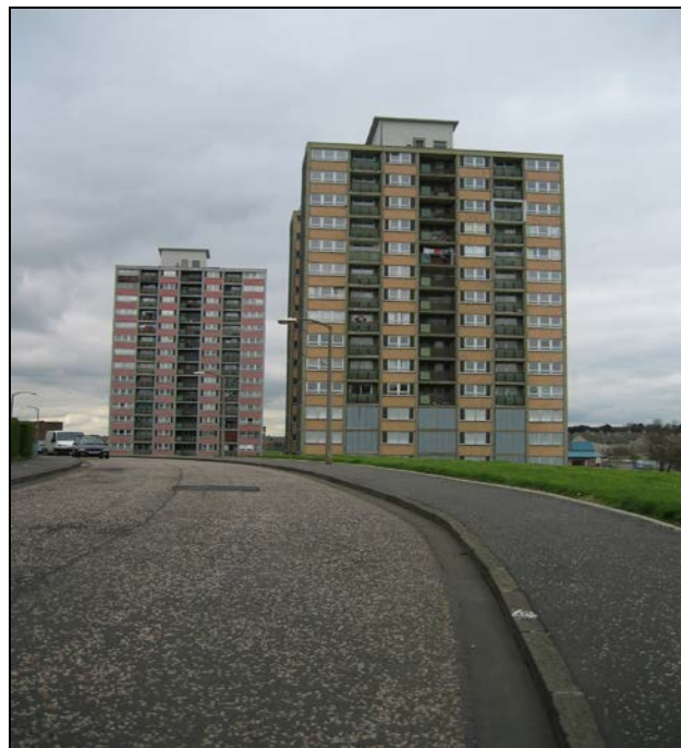
Allermuir and Caerketton Courts, due to be demolished later in 2005
