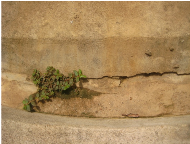
Figure 7 Plant growing through crack in well Figure 8 Severely eroded well casing apron
