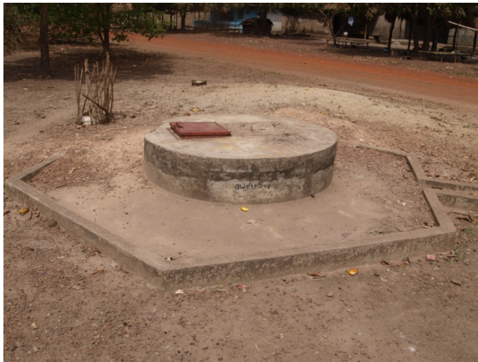
Figure 4 Masokoh Village Well
