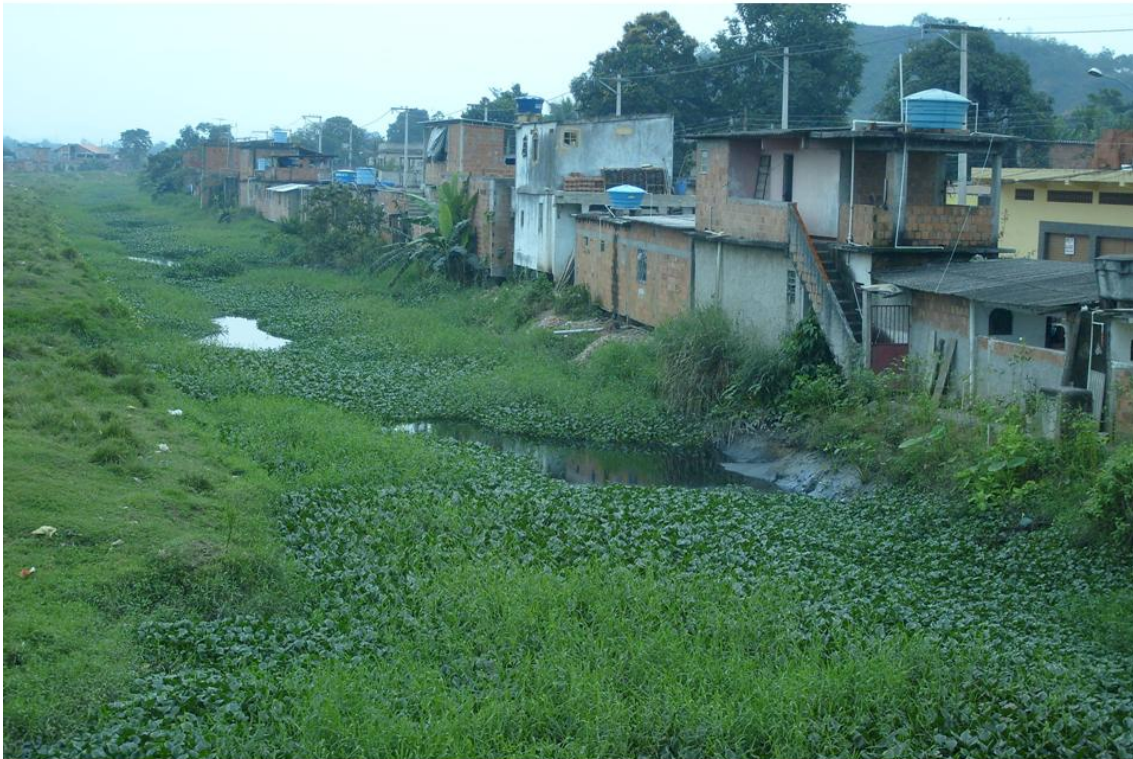
Figure 2. Houses built in the floodplain and along an abandoned drainage canal in the Iguaçu catchment.
