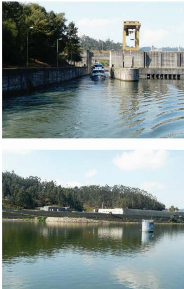
Figure 4 – Boat passage at the Crestuma-Lever dam and the Lever water treatment plant.
