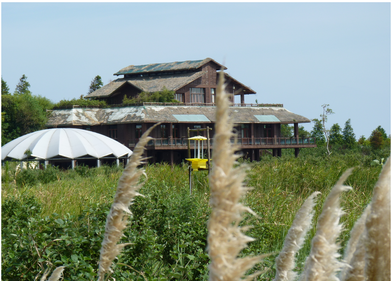
Visitors Centre, Dongtan, site of planned eco city on Chongming Island, off Shanghai 2012
