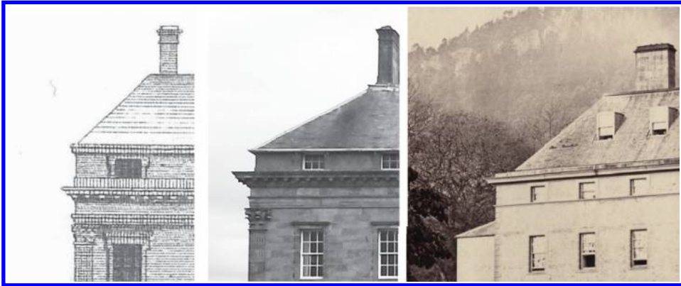
7. Kinross House, east facade, comparison of Vitruvius Scoticus plate 62 (left) and photograph (middle) showing the vanished masonry cornice gutter and attic windowcases. (Simpson & Brown Architects); Moncrieff House (right), in the nineteenth century, showing the masonry cornice gutter and attic windowcases lost at Kinross House. (Copyright: Perth and Kinross Council)
