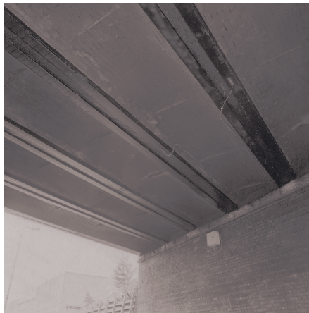
King Street Bridge, Mold
