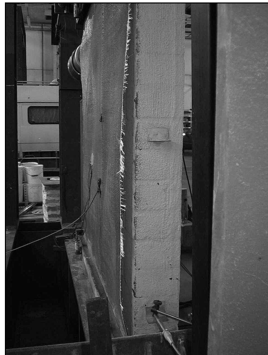
Figure 11 – De-bonding at opposite side to loading point (concrete 2)
