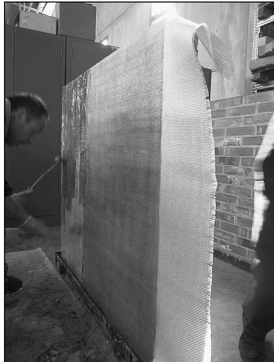
Figure 3 - Wet lay-up of glass-fibre reinforcement in epoxy resin
