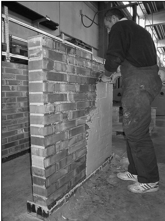
Figure 2 - Application of epoxy filler layer to clay wall
