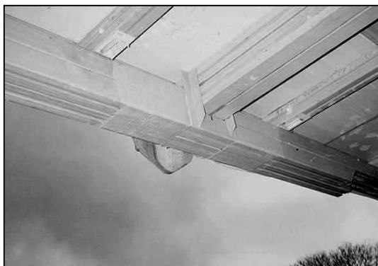
Figure 6: CFRP strengthening of the edge beam
