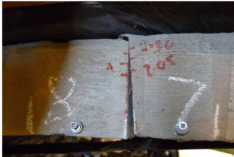
Figure 7. Mixed shear and flexural cracking failure at intrados crack (S-1) - viewed from the east
