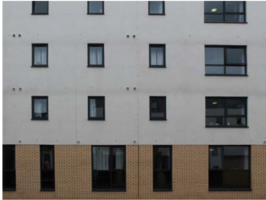
Fig. 8 – 9 Beaver Bank Place Inward-opening windows of c. 1825mm head and c. 1100mm sill allow for cleaning from within. NB: Fixed lights do not appear to comply with requirements of BS8213.
