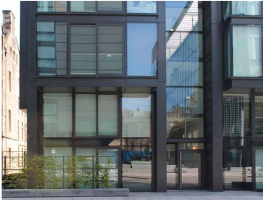
Fig. 4 – 5 Quartermile Fixed and sliding glazing not reachable from within, as per requirements of BS8213. Factoring contract required.
