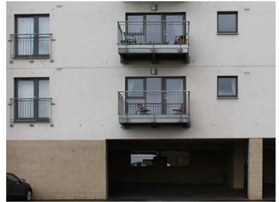
Fig. 10 – 11 Corinthian Quay Balcony allows head heights greater than 1825mm, and fixed glazing reachable from balcony.
