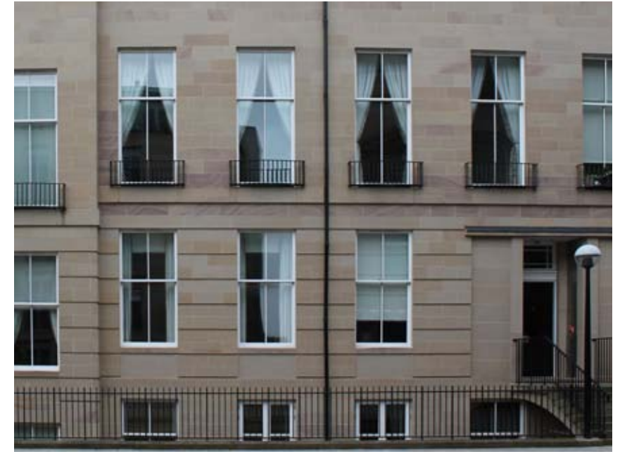
Fig. 6 – 7 St. Vincent Place Large vertically sliding and inward-opening windows. Upper sash does not lower to under 1825mm. Outer face not reachable within 556mm. Windows not cleanable as per requirements of BS8213. Factoring contract required.
