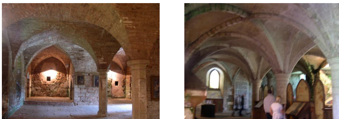
Figure 8: Lay Brothers' Block at Rufford Abbey (2007): Groin vaults at the cellars (left) and ribbed vaults at the adjacent frater or refectory (right)
