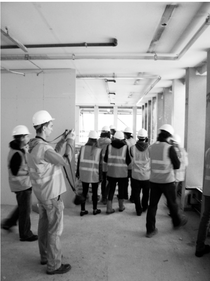
Fig 2 - Architecture students on a construction site visit at a university building refurbishment project [Photo: John-Paul Walker]
