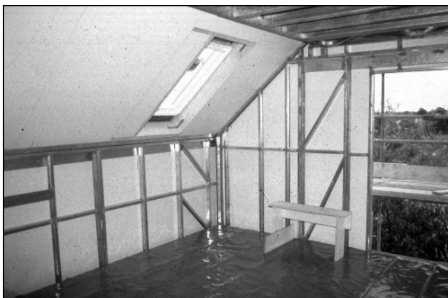
Figure 14. Open-roof system in the OBU house (kept open for demonstration purposes)
