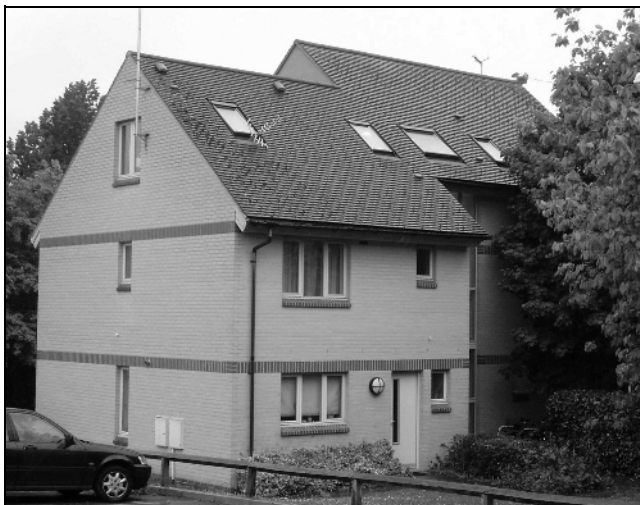
Figure 13. Oxford Brookes demonstration building constructed using light steel framing
