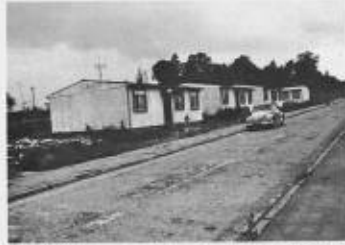
A. All the courtyard house tenants came from this nearby prefab estate; the row of prefabs shown here are a few of the ones left before demolition.
