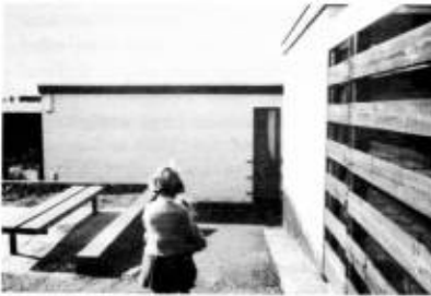
G. Looking towards the living-room south light window of house No. 16; protecting bars fitted across this window only encouraged children to climb up and peer through window.
