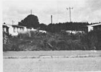
B. The backyards of the prefab houses provided little privacy from adjoining neighbours; note the large storage sheds referred to by tenants as 'cellars'.
