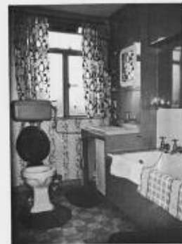
E. The prefab bathroom was well provided with built-in fittings; the courtyard house tenants complained that their new bathrooms seemed small in comparison and they disliked not having the wash hand basin boxed in; also missed was the heated towel rail.
