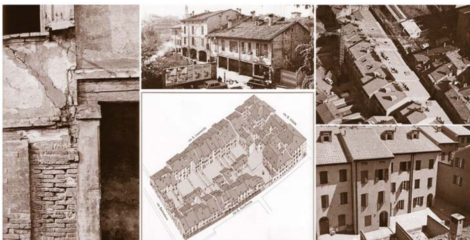
Bologna, 1975-85. Economical Popular Housing Plan (PEEP). Restoration of San Leonardo urban block.
