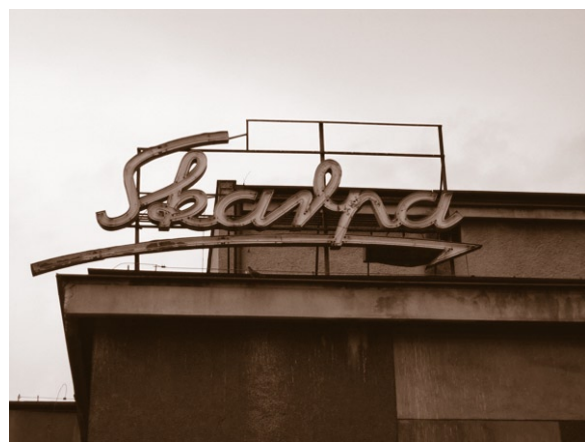
The front of Cinema Skarpa in 2008 shortly before its demolition. Photo: Ella Chmielewska
