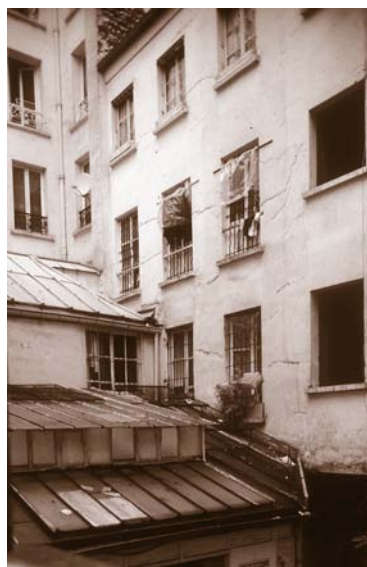
In Ilot operationnel 9/33 of the Marais, at the north-west side of the area, a complex plan of 1969 for radical surgery to internal courtyards was scrapped in 1976, leaving internal courtyards such as this one, north of the rue des Gravilliers, more or less intact. (M. Glendinning, 2009)
