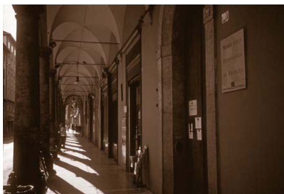
Exterior of the former S. Mattia Convent, Bologna, a 'large container' converted into a range of community uses including a Museum of the Resistance. (M. Glendinning, 2008)
