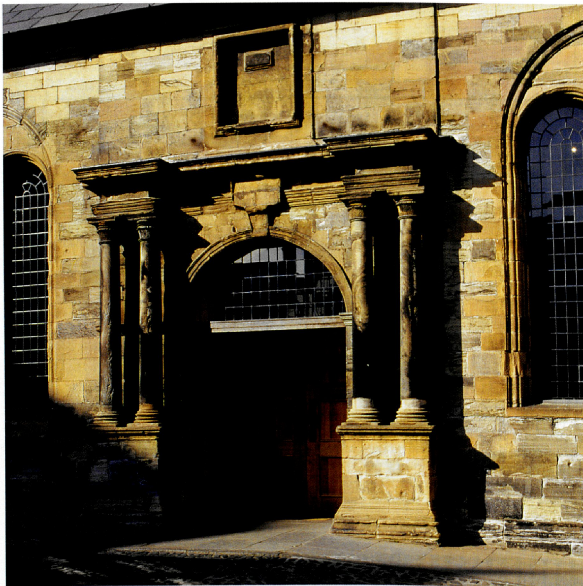
Fig. 5. Chapel Royal, detail of principal entrance (© Historic Scotland, c. 2000)
