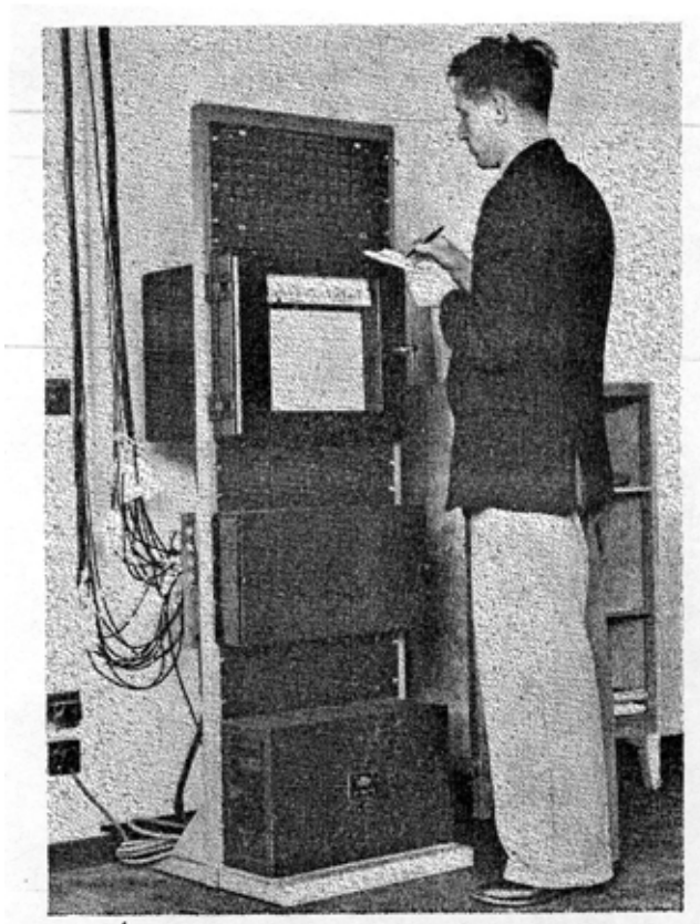
Figure 4: Central recording device used in heating experiments at the BRS
