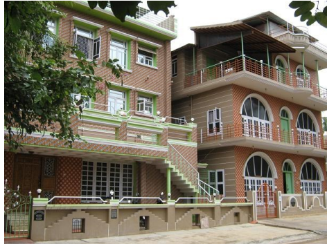
Fig.3: View of Contemporary Housing pattern
