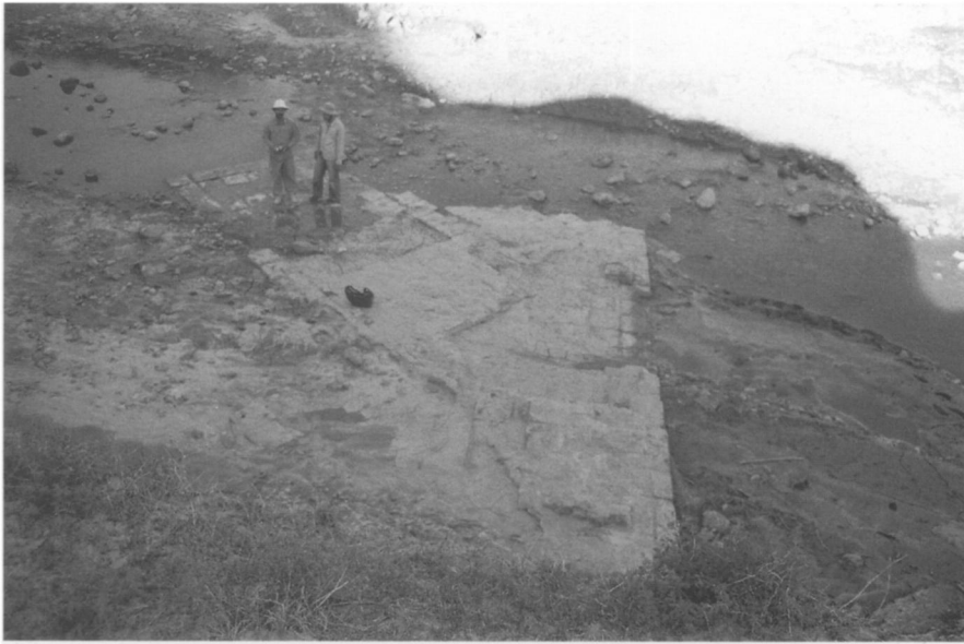
Fig. 14. Feature of Gorgan Wall bricks at east end of wall between Fort 2 and 2A. (See Fig. 13 for its location.)
