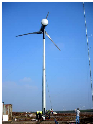
Figure 8: Installation of 15kW C-GEN prototype at Myres Hill wind farm
