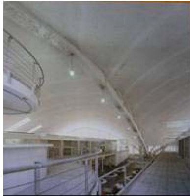
Figure 1. The deep rib reinforcing the intersection of the main conoid vaults, City Market, Pola de Siero (1930)
