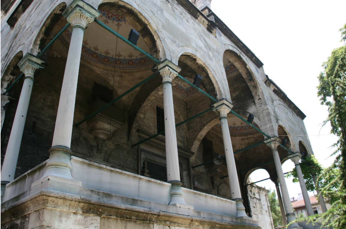
Figure 240. Ayazma Mosque, entrance portico.
