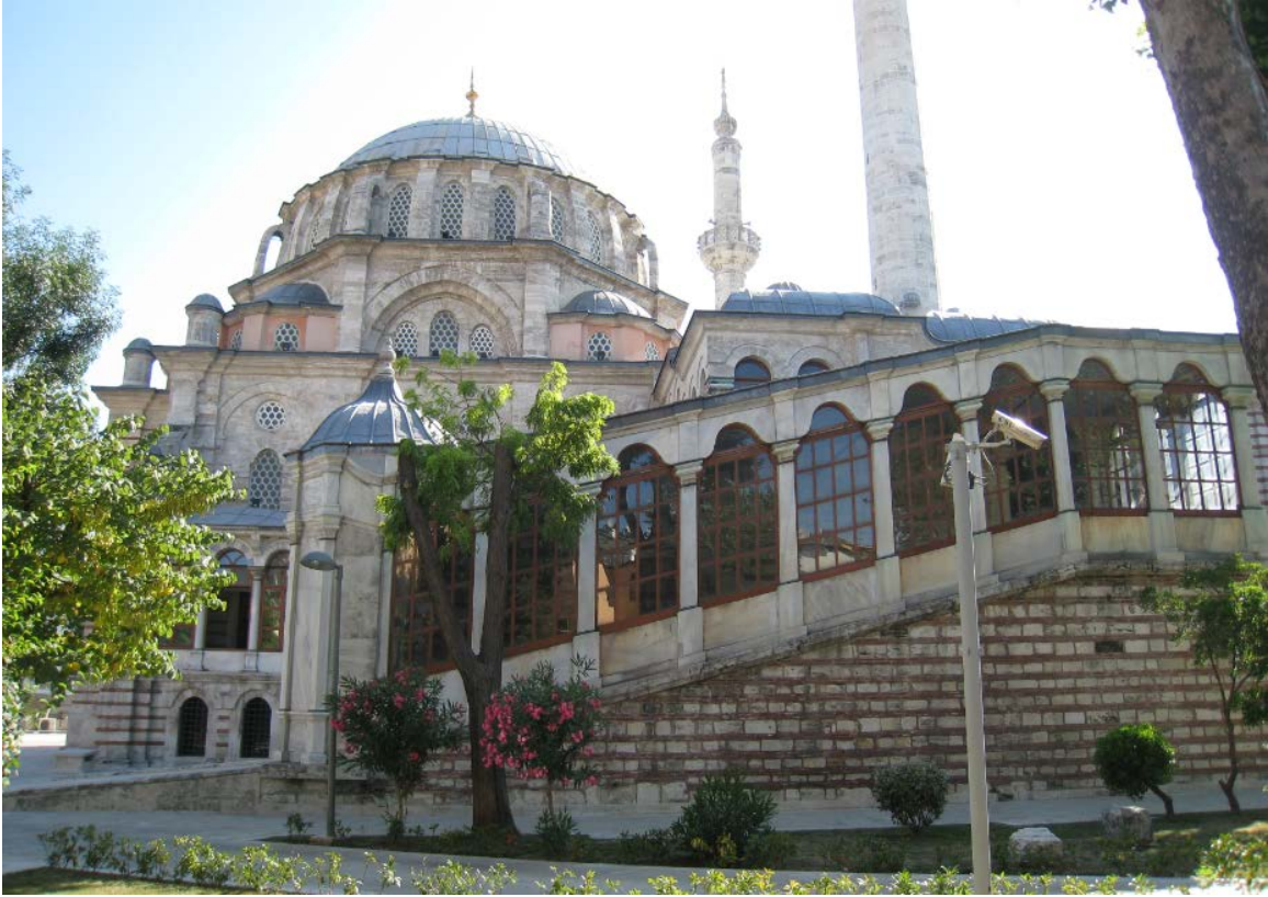
Figure 283. Laleli Mosque, looking towards the sultan's pavilion.
