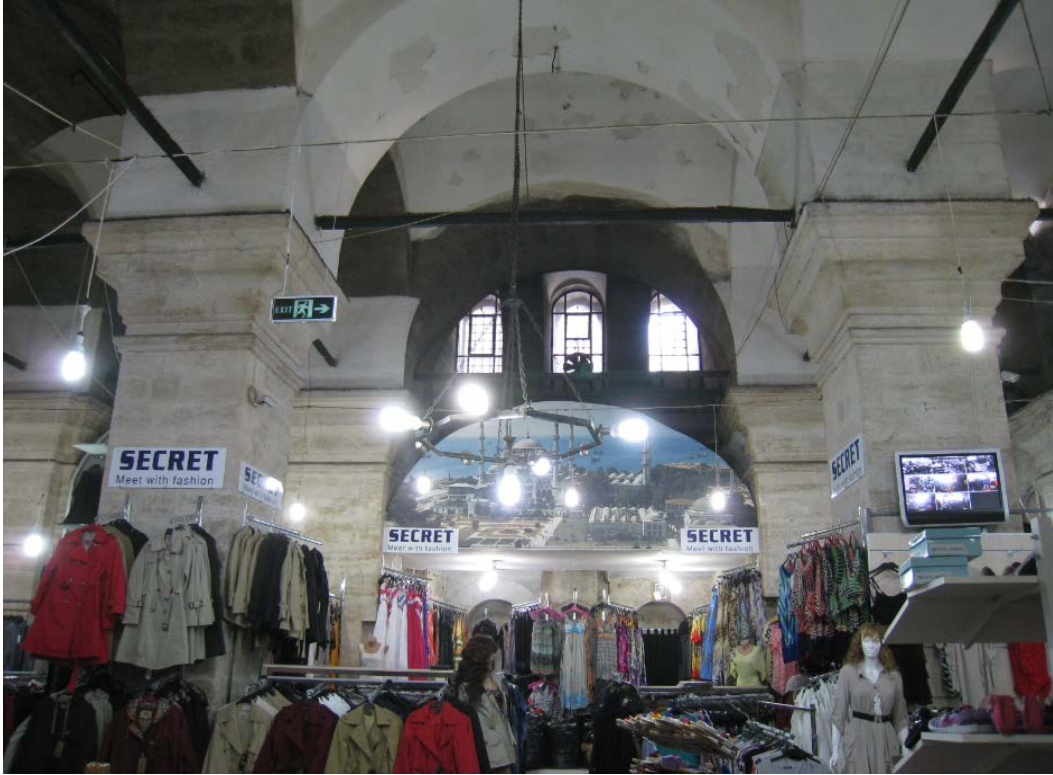
Figure 277. Laleli Complex, vaulted basement.
