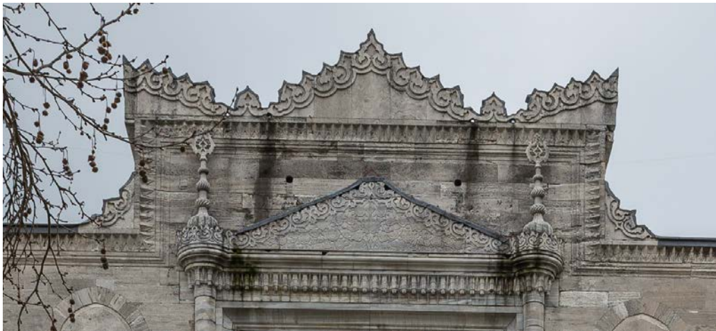
Figure 257. Süleymaniye Mosque, pinnacles and cresting of the courtyard gateway. © Arild Vågen / Wikimedia Commons.
