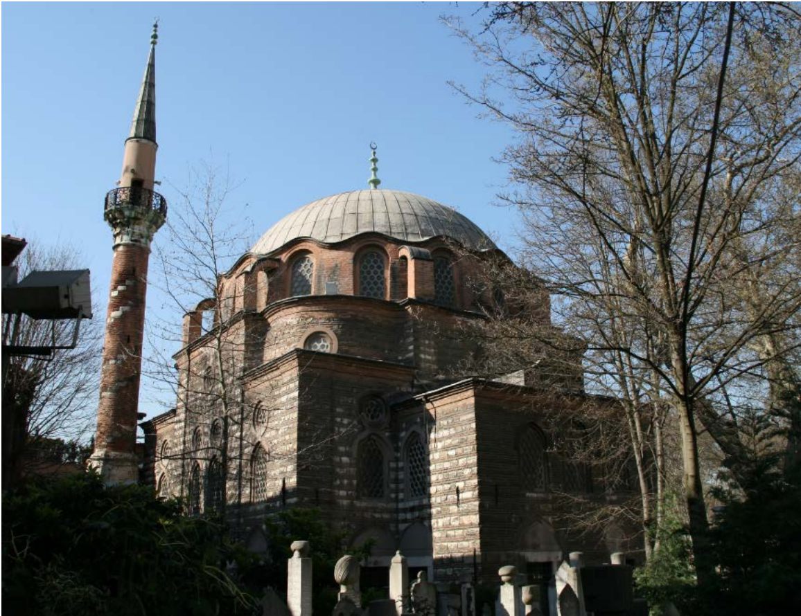
Figure 320. Zeyneb Sultan Mosque, Istanbul, 1769.
