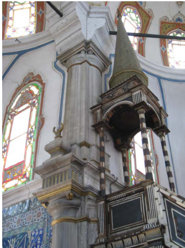
Figure 412. Beylerbeyi Mosque, cap of the minbar and the adjacent pier.
