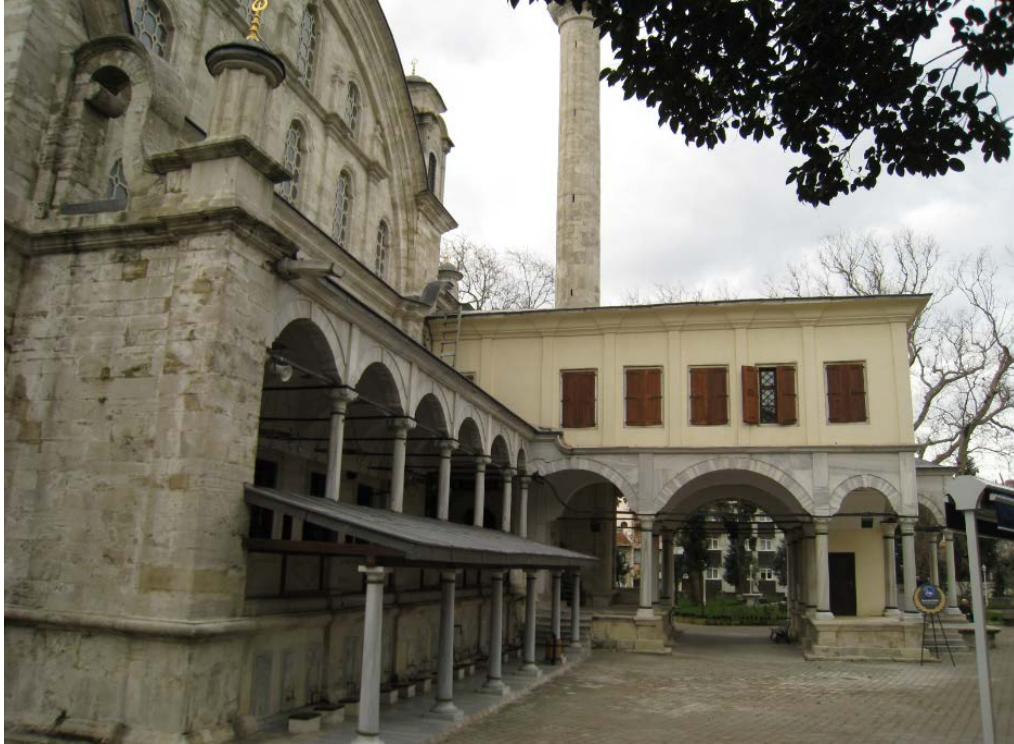
Figure 455. Selimiye Mosque, looking towards the northeast wing of the sultan's pavilion.
