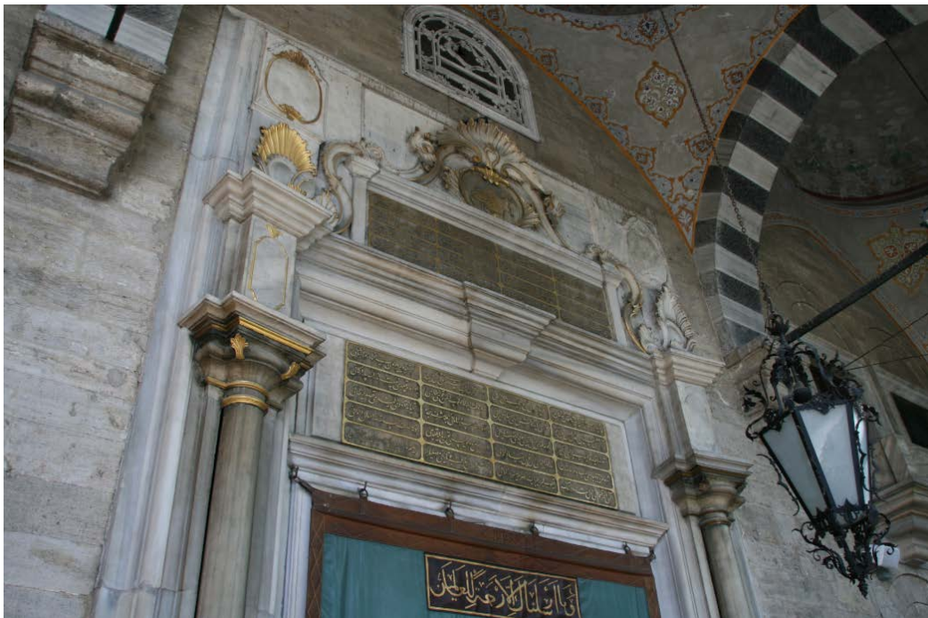
Figure 443. Eyüp Sultan Mosque, main entrance.
