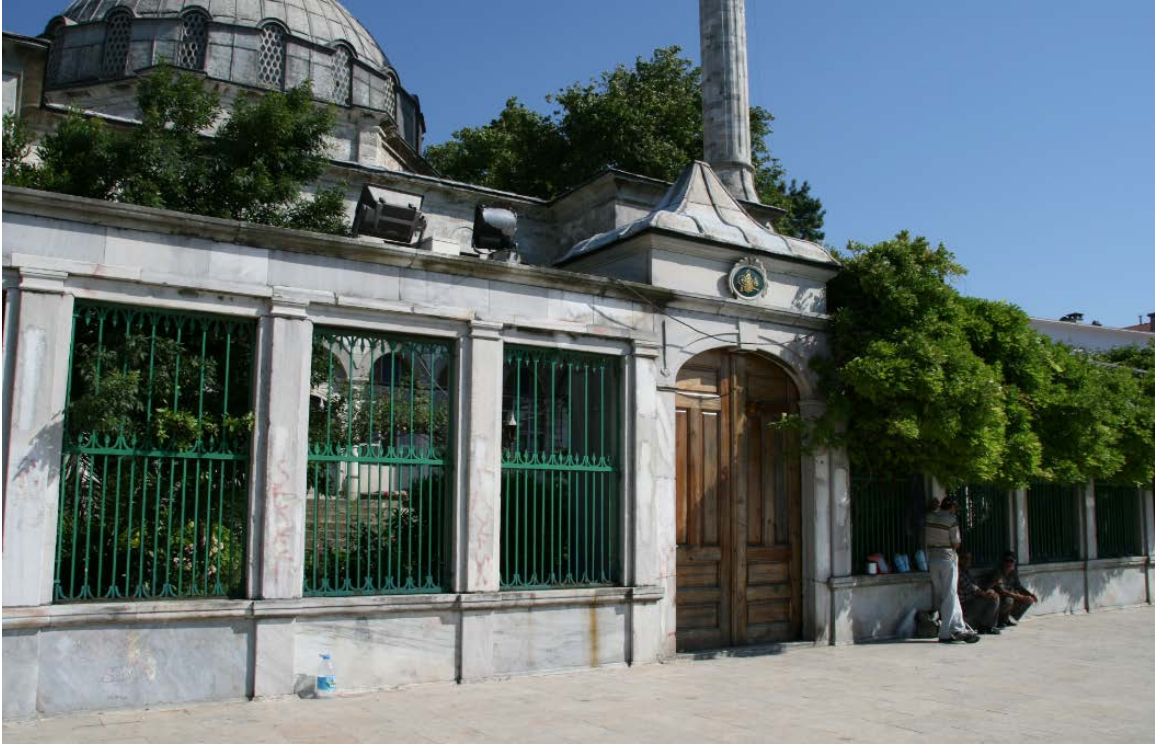
Figure 428. Beylerbeyi Mosque, rebuilt perimeter wall and gate, 1810–11.
