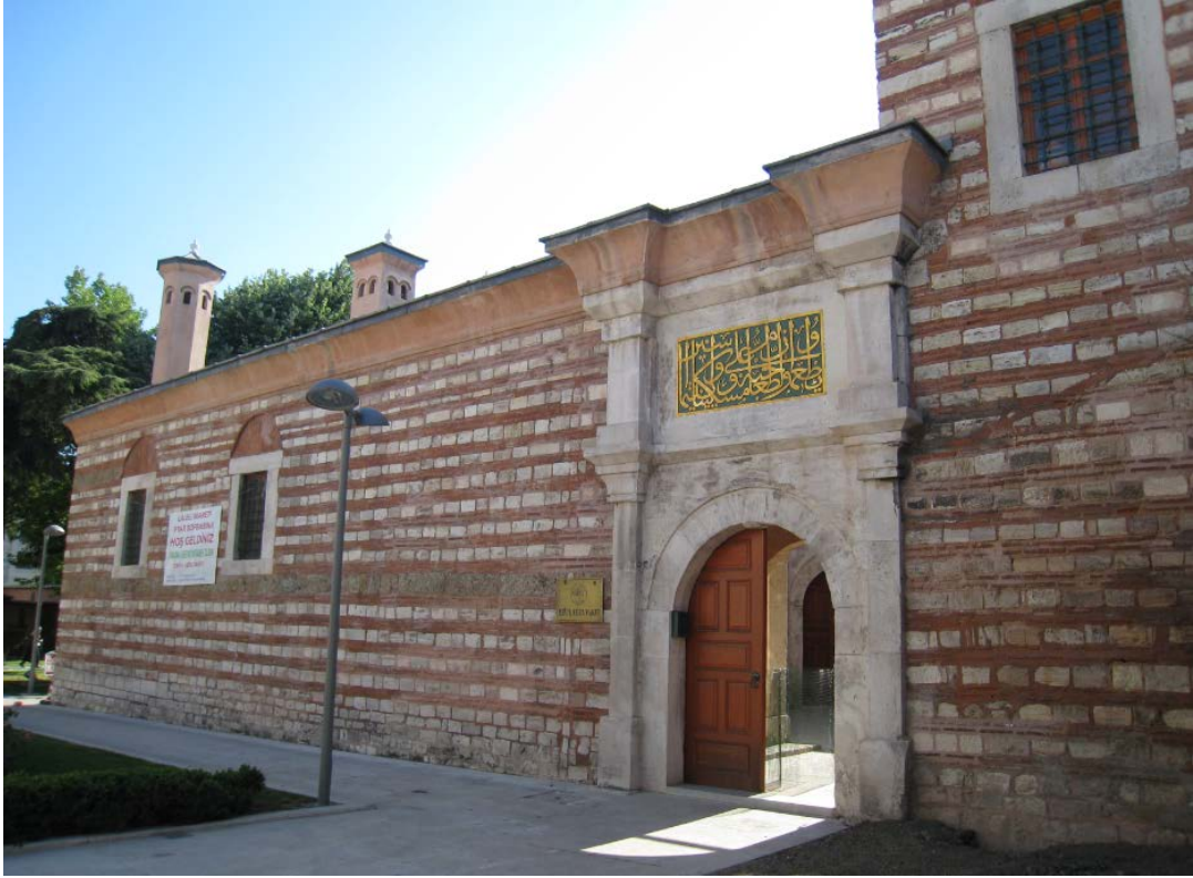
Figure 275. Laleli Complex, imaret, facade.
