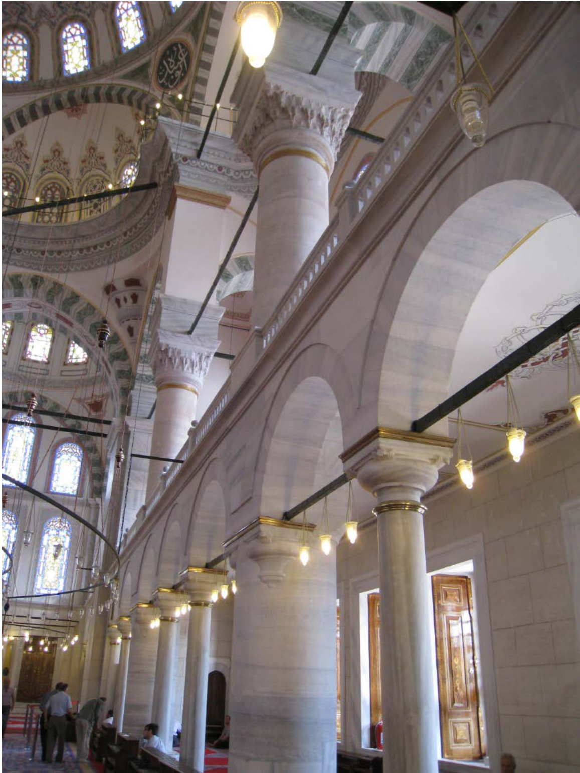
Figure 354. Fatih Mosque, lateral gallery, showing the muqarnas capitals of the piers and the scroll capitals of the columns.
