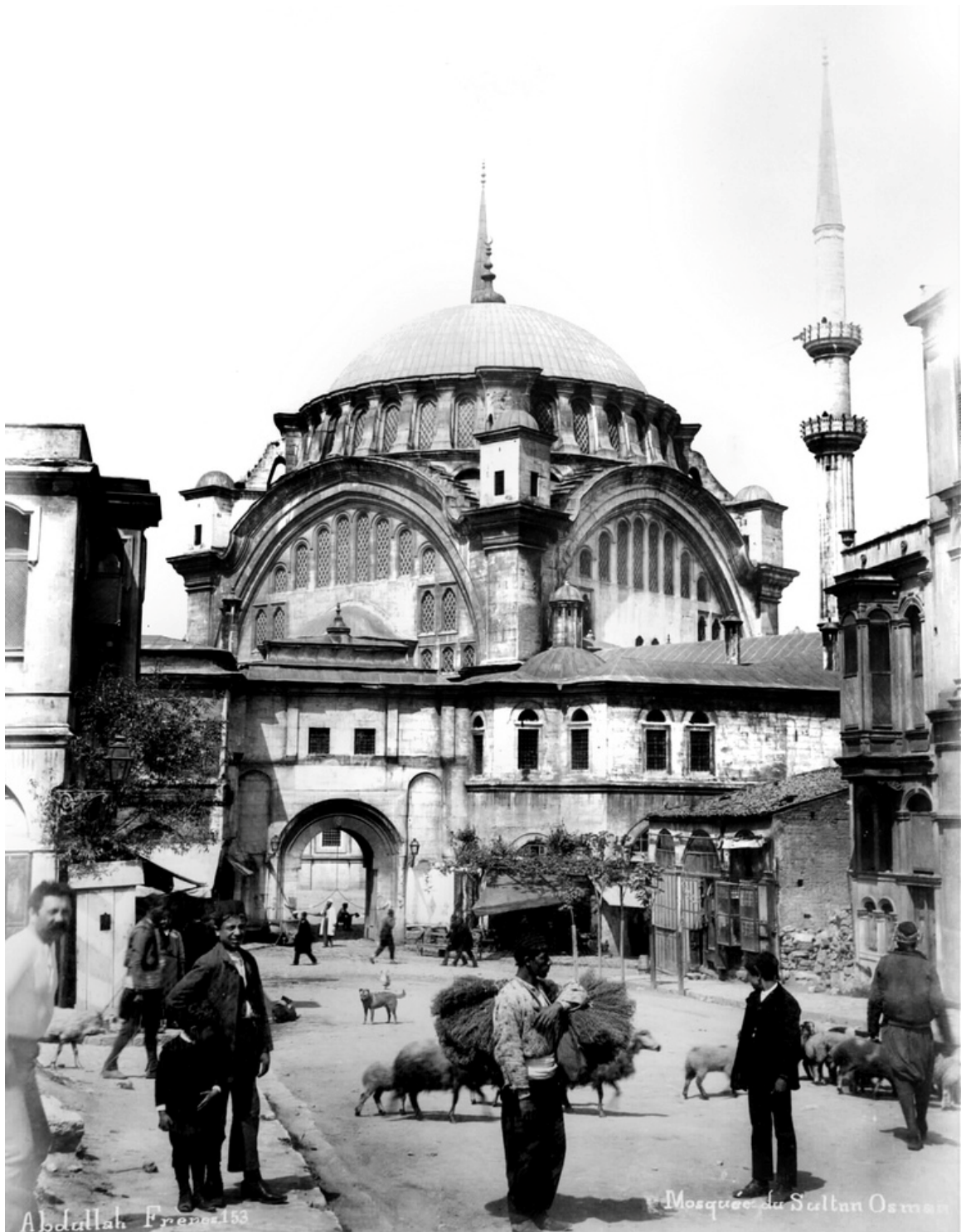
Figure 123. Photograph by Abdullah Frères of the Nuruosmaniye, taken from in front of the east gate and showing the original form of the minarets, pre-1890.
