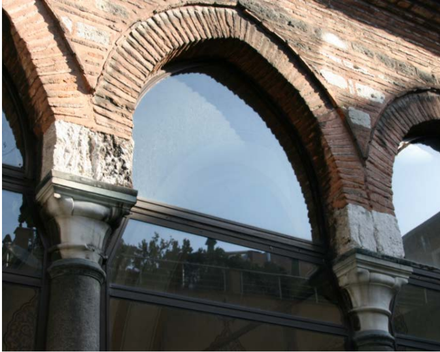
Figure 322. Zeyneb Sultan Mosque, arches and column capitals of the entrance portico.
