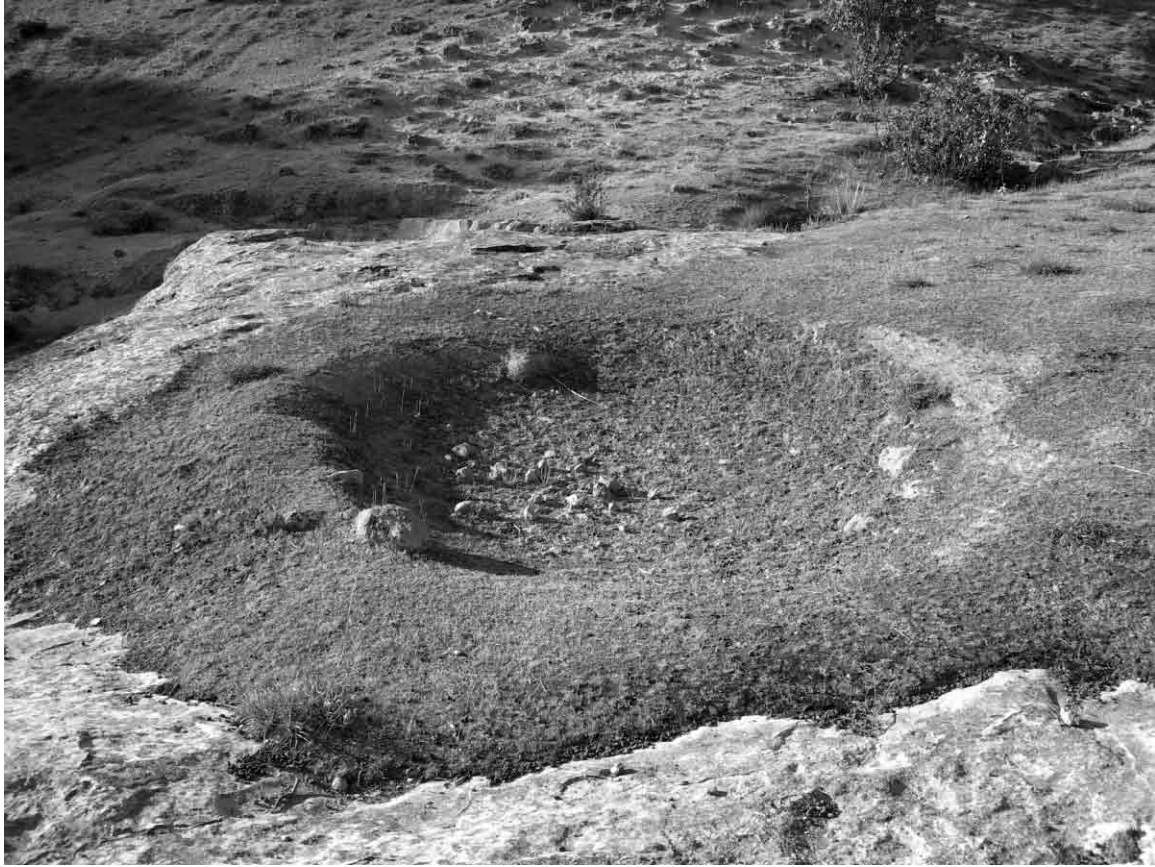
Figure 9. A small earthen check dam at Site 91. The reservoir is 1.5 m in diameter.
