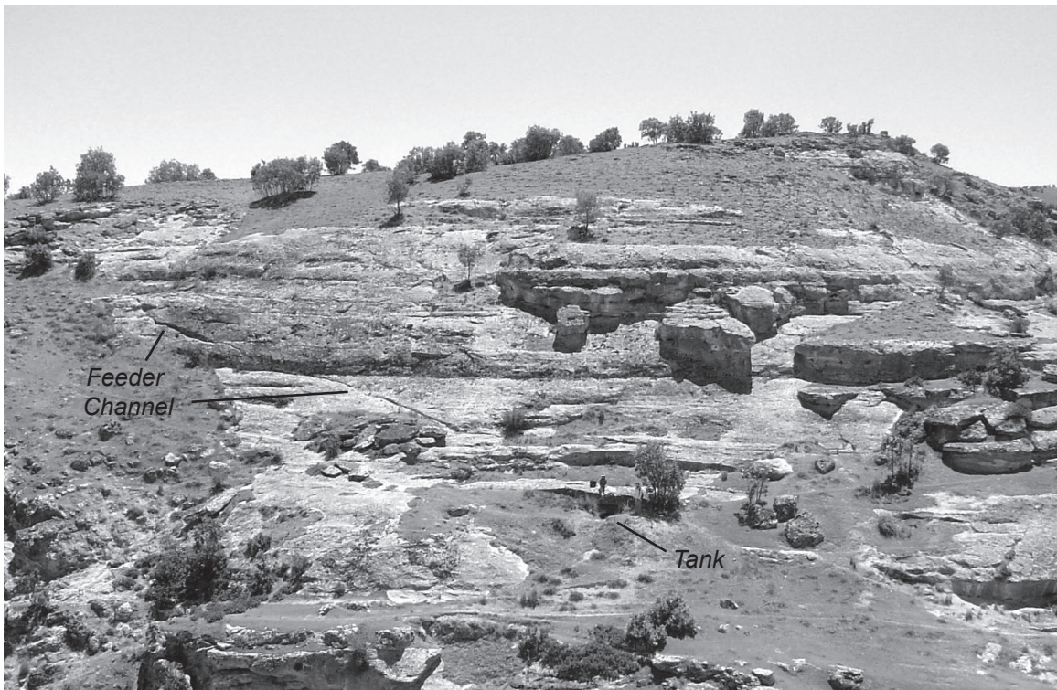
Figure 10. The large cistern at Site 37, facing east. The entrance to the tank is near the figures at center; the feeder channel runs diagonally from the upper left down to the tank.
