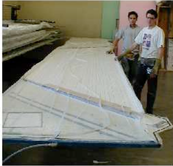
Fig. 13. Scintillator strips and manifolds being vacuum bonded (laminated) to the bottom aluminum cover.
