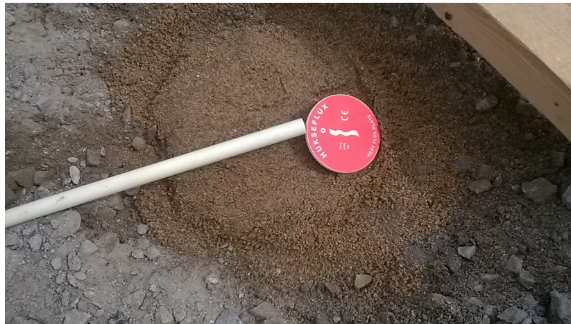
Figure 2. Installation of heat flux plate “Hukseflux” before asphalt pavement.
