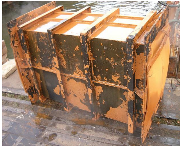
Figure 8. A box girder that was initially corroded in real sea water conditions from which the specimens for the tensile strength tests were cut from (Saad-Eldeen et al., 2011).
