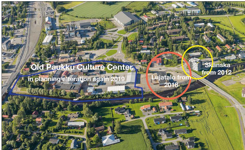
Figure 6. Old Paukku Culture Centre is again under planning alteration in 2019, because Lapua town aims to terminate the conservation conclusion of the Canteen (conservation ordered by Ministry of Environment). Source: City of Lapua. On the eastern part the high-rise plots are now in the area "not important to preserve", in the cultural heritage inventory the contract with Skanska was signed in 2012 and the building is completed and almost all apartments sold. Lujatalo is currently finalizing one eight-floor building and starting another, not as high.
