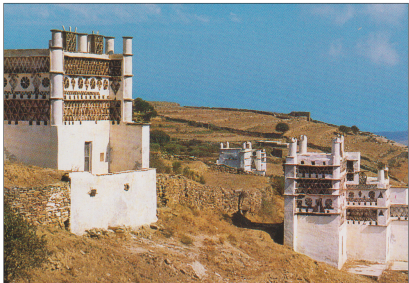
Figure 6. Dovecotes in Tinos hinterland (author's pic. archive).
