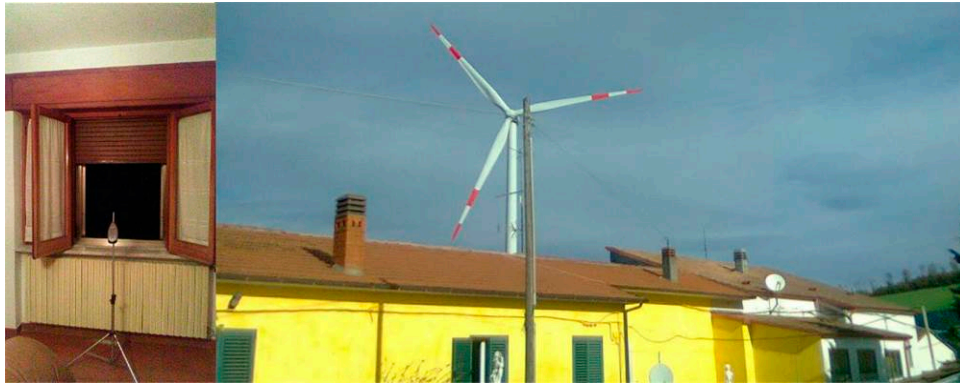
Figure 2. Equipment during the acoustic measurement process (on the left) and a view from the window of the house where it is clearly possible to identify one of the 4 turbines (on the right).
