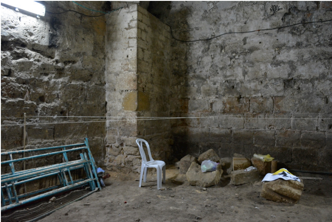
Figure 6: Strings connecting triangulation points
