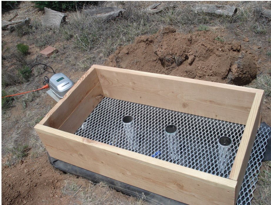
Figure 2-8 Partial nitrification planter installation.
