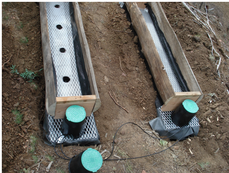
Figure 2-2 Planter Installation.
