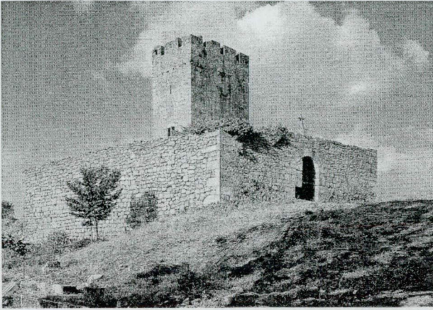
Figure 3 – Longroiva (North-East of Portugal): the keep and visible putlog holes to support the hoarding
