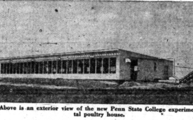
Above is an exterior view of the new Penn State College experimental poultry house.
