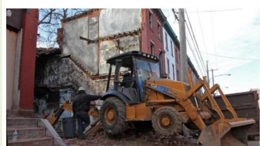
Workers demolish a North Philadelphia rowhouse. (Emma Lee/WHYY)
