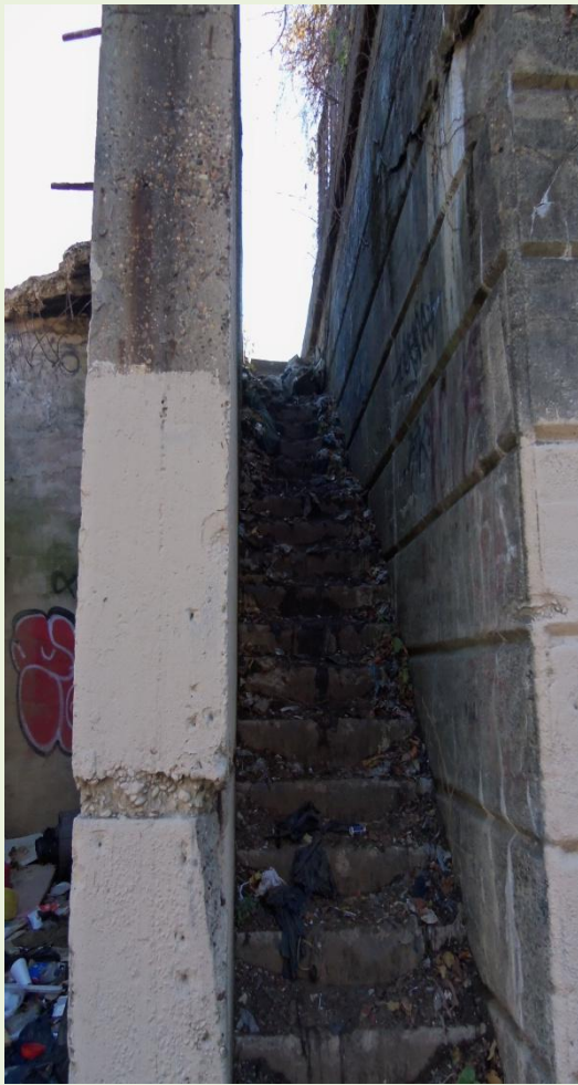
Stairs to viaduct from Emerald Street
