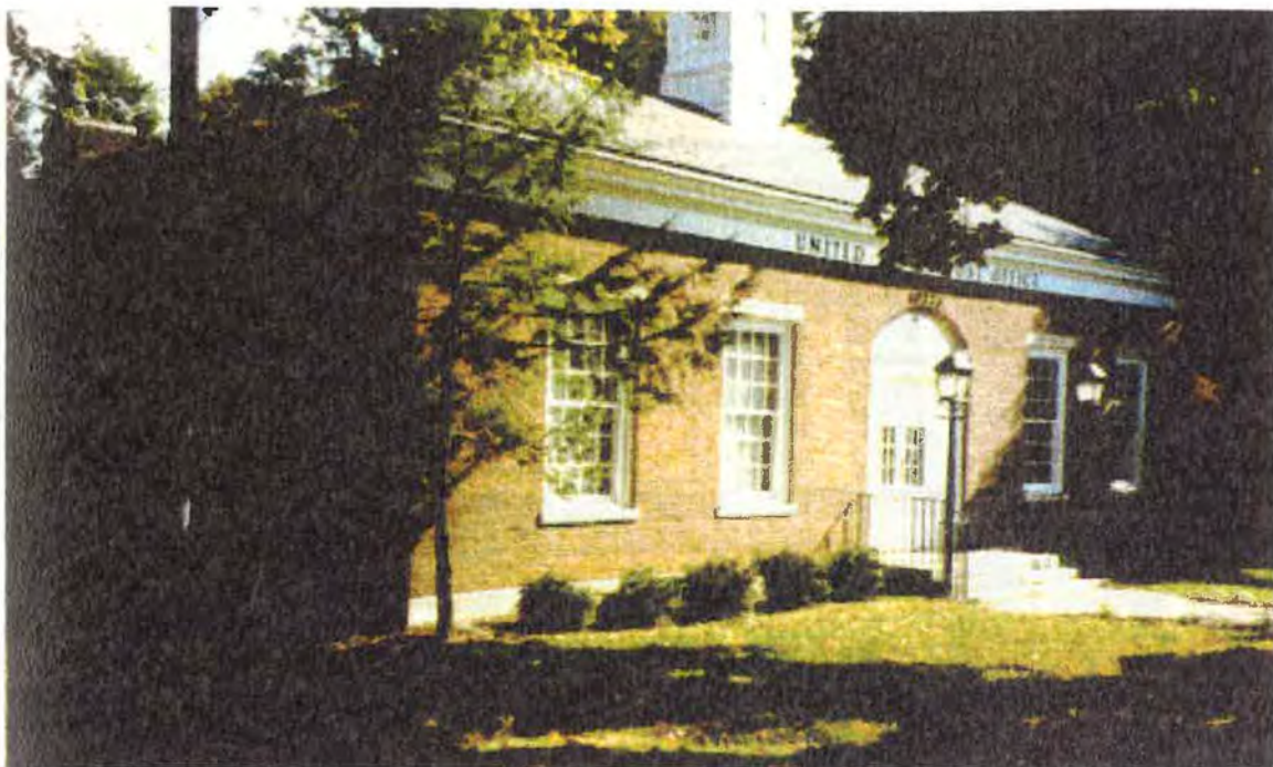
Figure 1. Anchorage. Exterior View of Post Office
