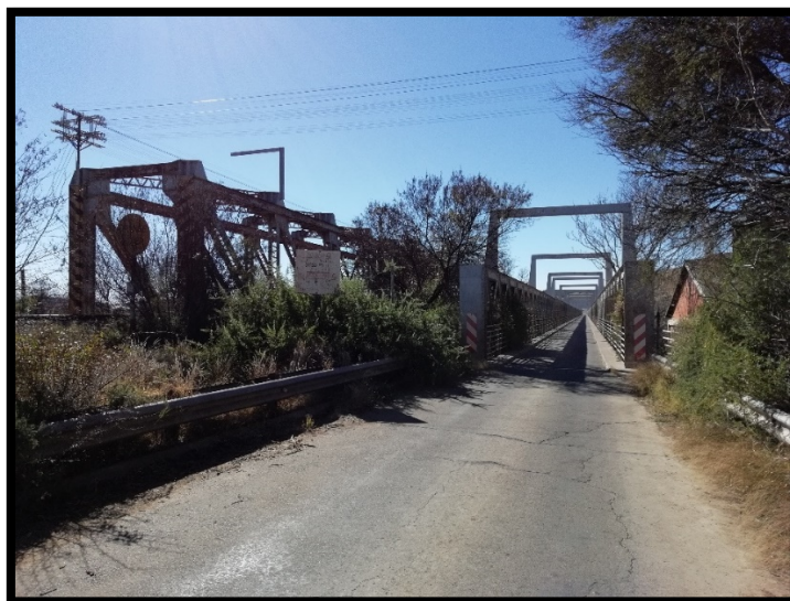
Picture 10: Orange River Bridge
