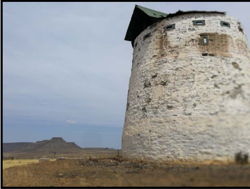
Picture 15: Blockhouse, Hospital Hill
