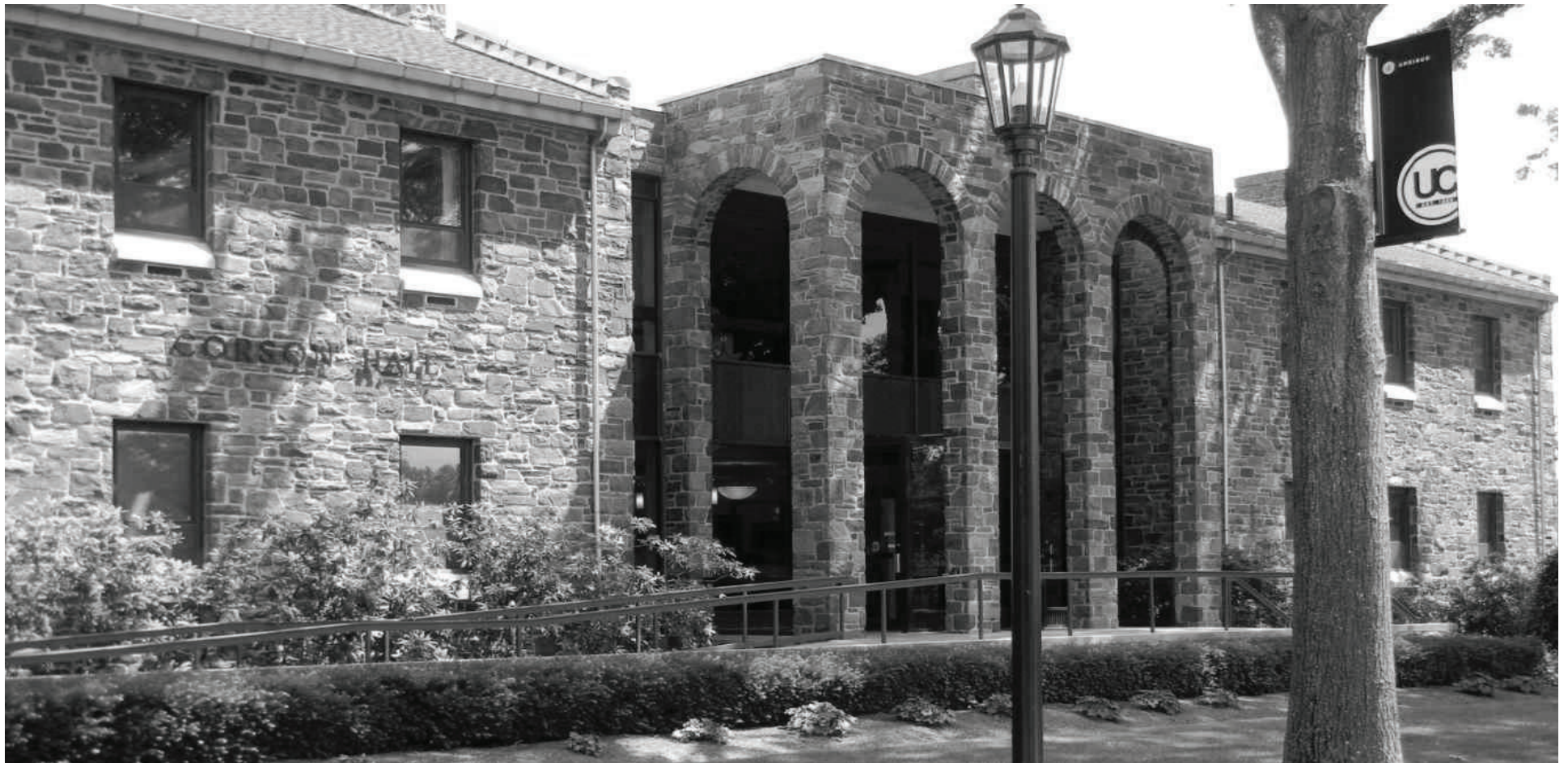
Corson Hall houses the business office at Ursinus.
