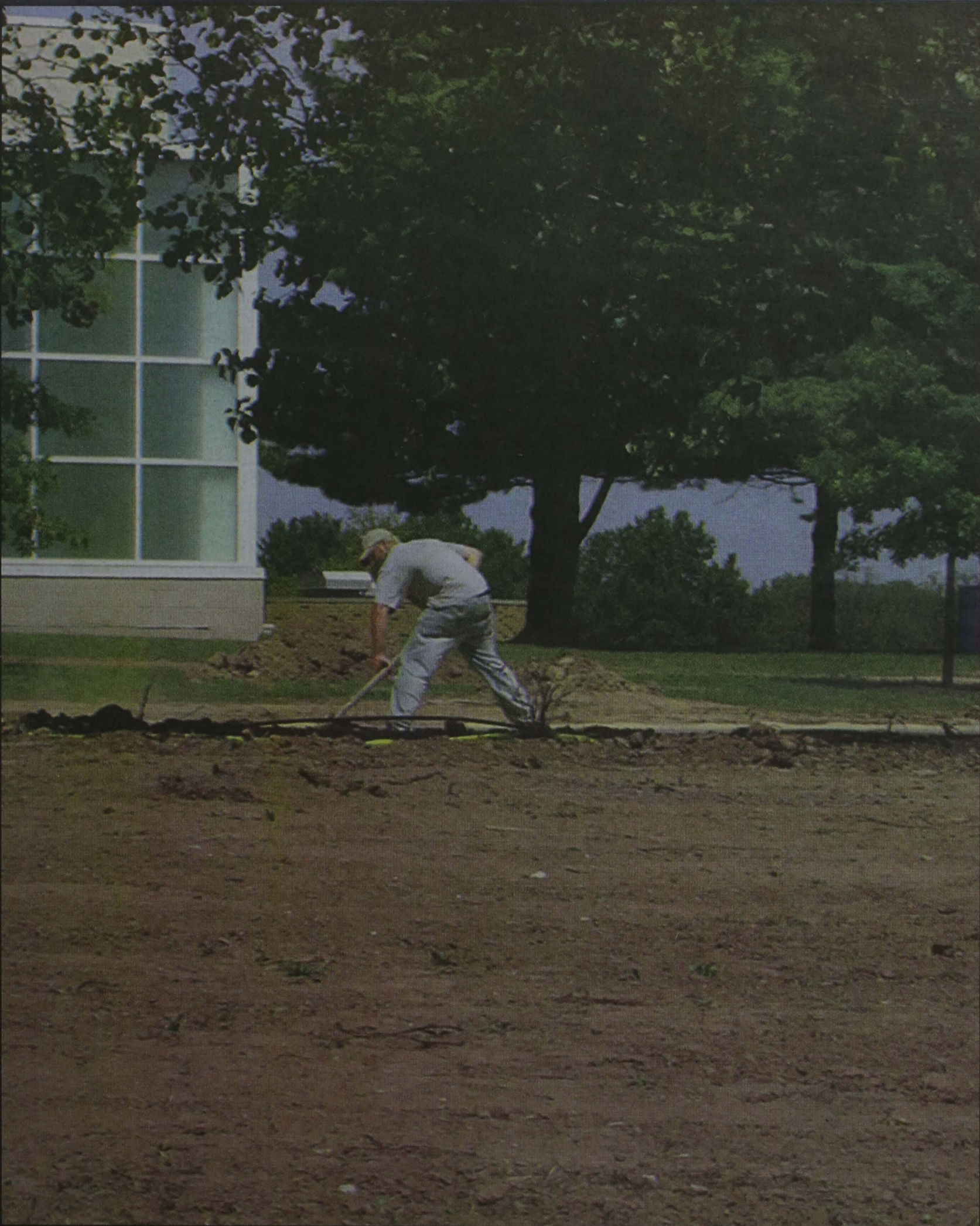
Construction Continues on Campus
