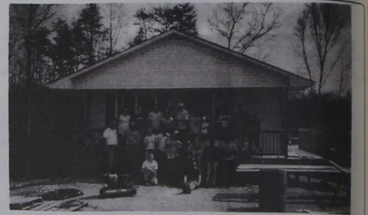
The ASB Club with workers from Habitat for Humanity in front of the home they helped construct. Staff Photo by Emily Callaghan
