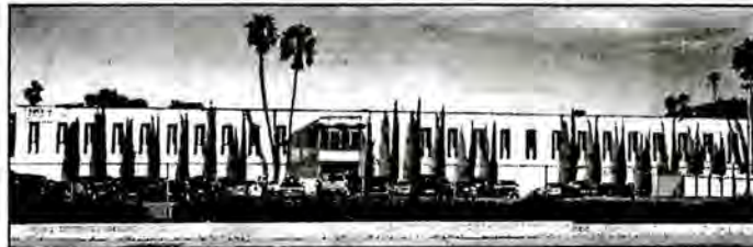
An industrial facility on Greenfield Drive in El Cajon is the site where, in the late 1980s, regional water board officials documented leaks in a chemical waste tank. Nancy E. Lewis / Union-Tribune
