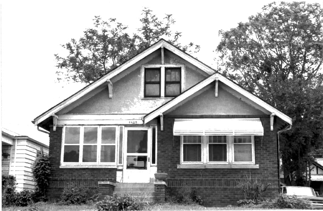
Fig. 2.17. Short sidewalls on one-and-one-half-story bungalow
