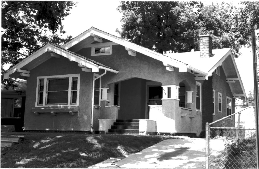
Fig. 2.8. Double gables on front facade
