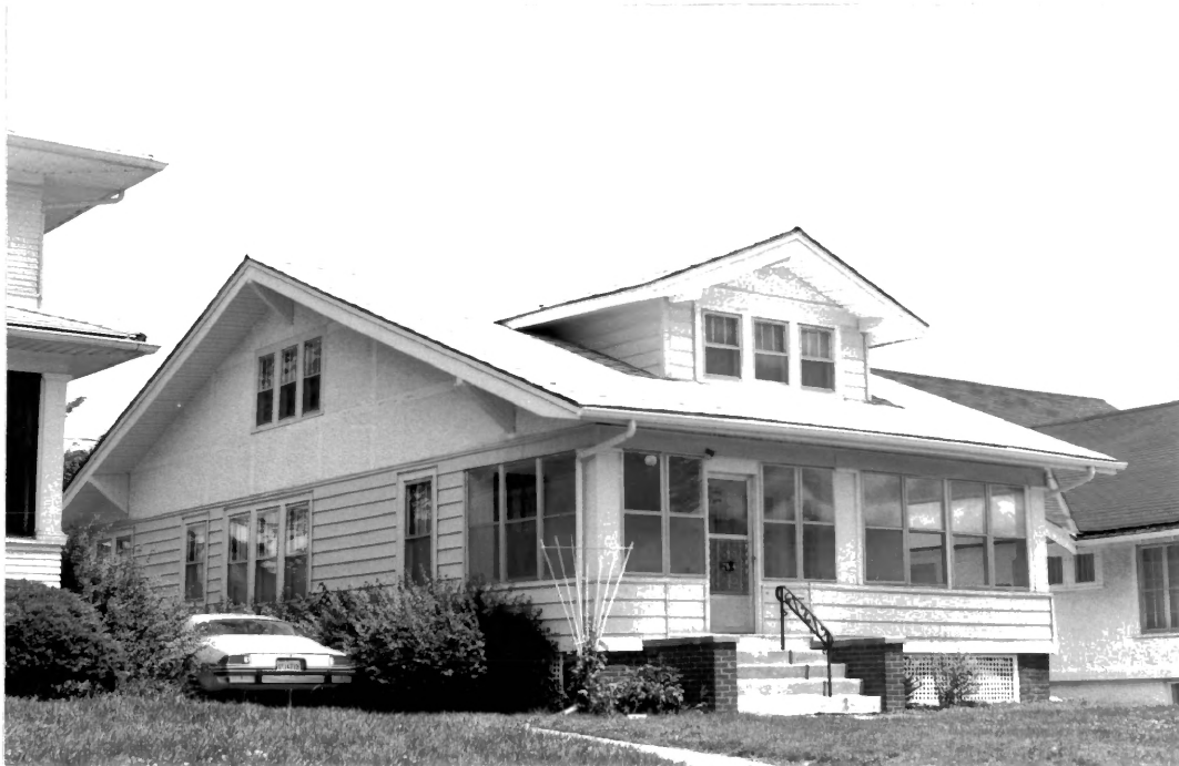
Fig. 2.26. Porch under main roof
