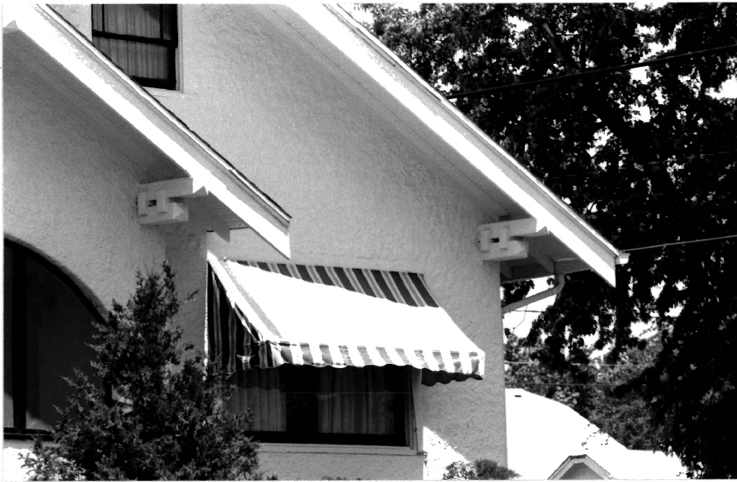
Fig. 2.6. Support brackets and visible rafter ends
