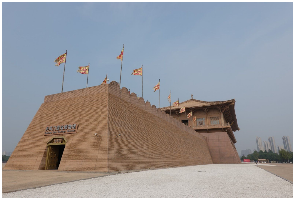
Figure 2.28 Danfeng Gate Heritage Museum, entrance, Xi'an, Shaanxi, China, 2019.
