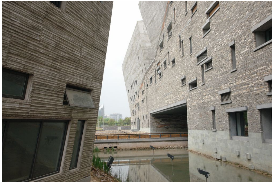
Figure 3.4 A water pond between buildings. https://www.gettyimages.com/detail/photo/ningbo-museum-of-art-view-the-water-platform-royalty-free-image/627846930 .
