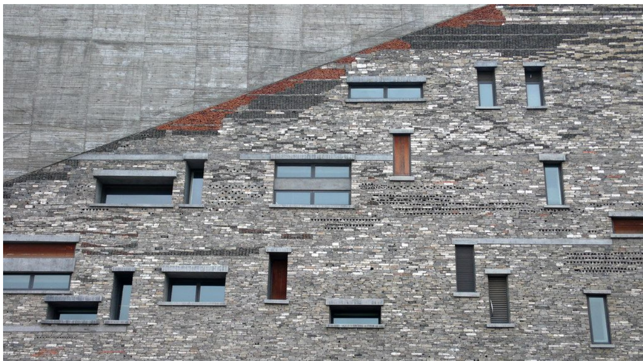
Figure 3.3 (below) Ningbo Museum, detail of the facade, https://www.pinterest.com/pin/114138171779249197/?lp=true .
