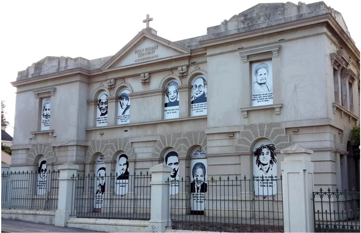
Figure 8. Completed project after installation at Holy Rosary Convent, 2015.
