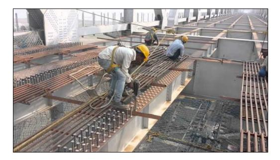
Figure 67: Drawn Arc Stud Welding [54]
