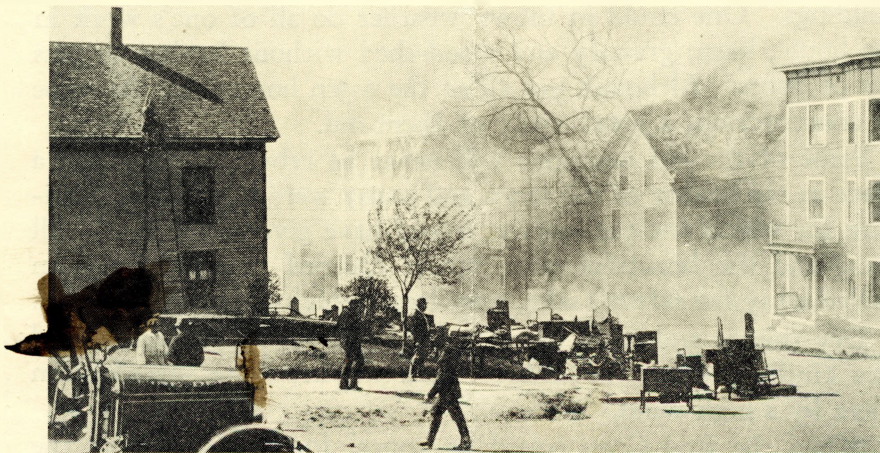
Fighting the flames at Auburn
